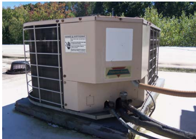
5: Split system condensing unit on roof
