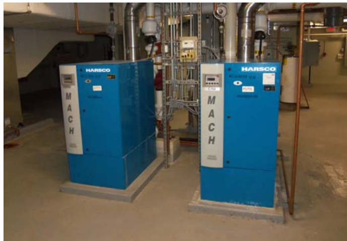
2: Hot Water Boiler Plant
